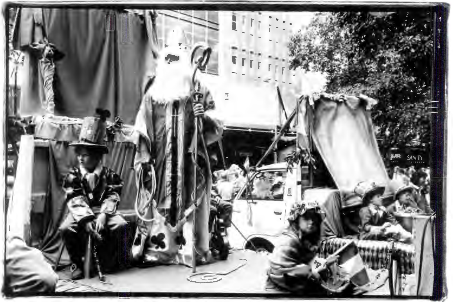
Casting out snakes from the shopping Mall. Melbourne March 1997.
